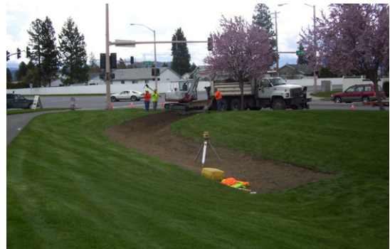
Grassed swale construction Source: City of Coeur d'Alene, Idaho
