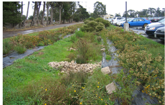
The use of vegetated swale along a surface parking lot Source: University of California, Santa Barbara
